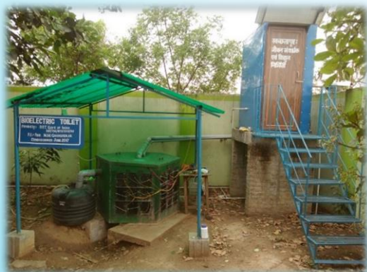
1500 litre field scale bioelectric toilet at IIT Kharagpur
